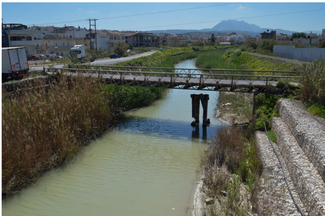
An old iron made bridge at the area of river run off.
