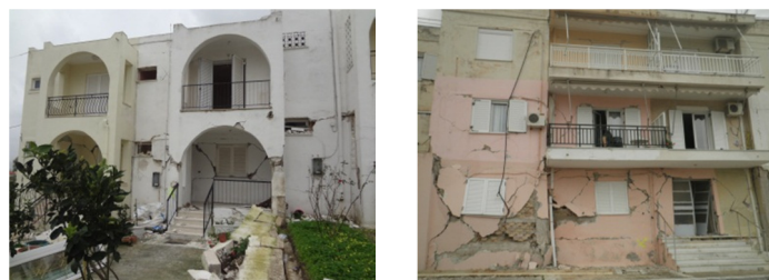
Figure 8: Public housing complex heavily damaged buildings in Lixouri.
