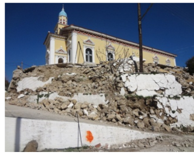
Figure 4: Failures at the stone retaining wall in Havriata village
